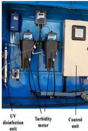
Figure 21: Inside the case of GMMW trailer
