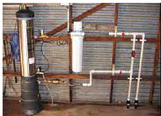
Figure 29: Ultrafiltration unit with prefilter
