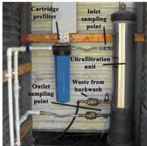
Figure 31: Ultrafiltration unit on property outside of Dadswells Bridge
