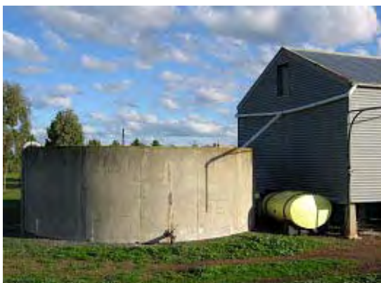
Figure 28: Feed water tank
